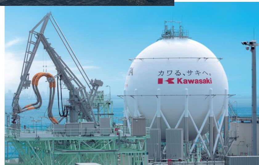
Liquefied hydrogen storage tank
