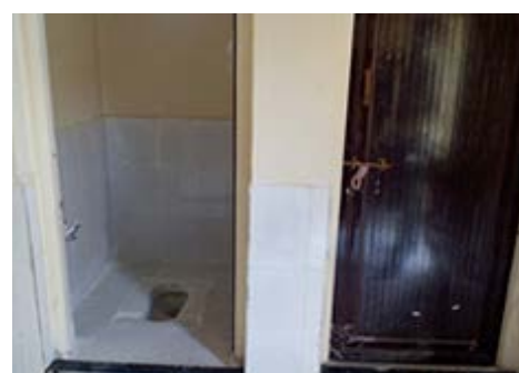
Toilet at Bolegaon Village
