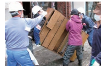
2 Earthquake disaster area support volunteers (Iwate Prefecture)
