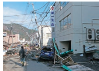
Kamaishi Unit Office immediately after the disaster
