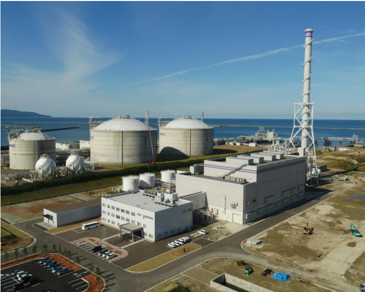
▲ Joetsu Thermal Power Station in Joetsu, Niigata (photo courtesy of Tohoku Electric Power)
